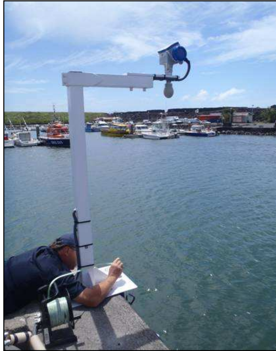
Fig.7: Installation of the tide Gauge of Sainte-Marie (La Réunion Island) for Tsunami warning.
