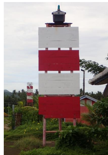
Figure 72: Aleipata Leading beacons (rear beacon light missing)
