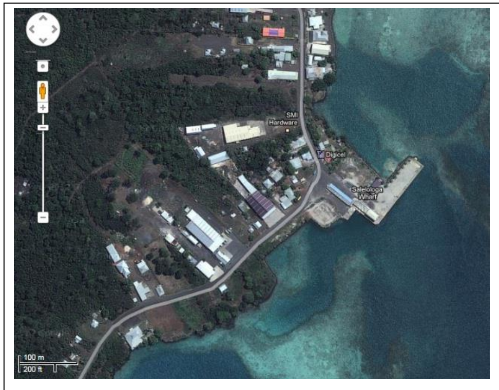
Figure 63: Salelologa Wharf (Source: Logistics Capacity Assessments)
