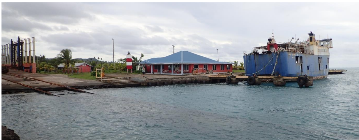
Figure 70: Aleipata Port – slipway, front lead, terminal & wharf ( Lady Samoa II being dismantled)
