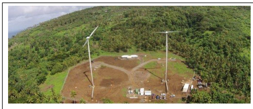
Figure 46: Wind Farm – Vailoa Aleipata, Upolu (Source: Energy Matters)
