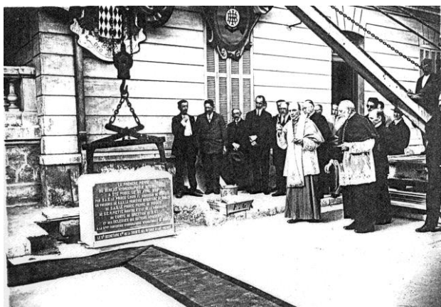
Laying the foundation stone - 20 April 1929
