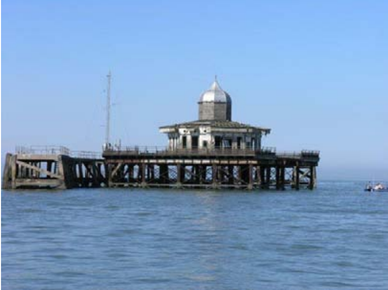
Isolated seaward end of Herne Bay pier
