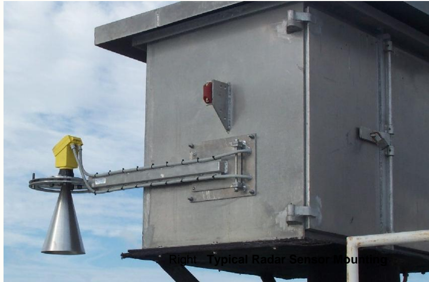
Typical Radar Sensor Mounting Environmental Protection Agency
