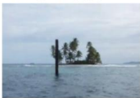
A buoy marker with missing topmark
