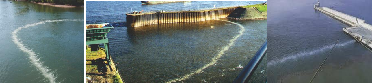
F29.2, "Oil retention barrier (high pressure pipe)"
