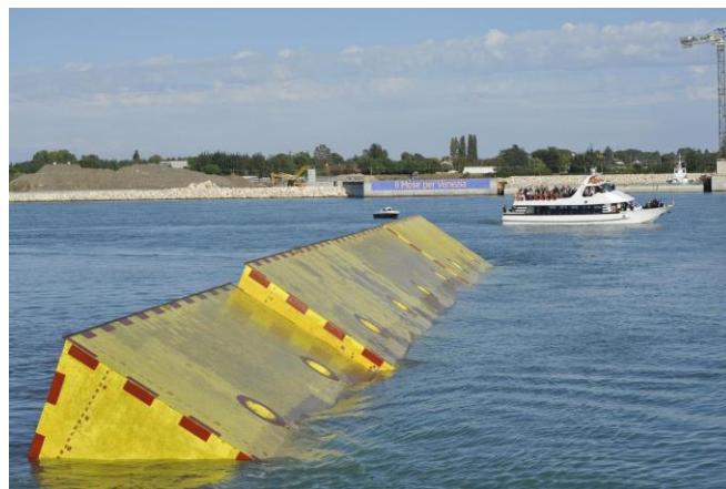
Venice Flood Barrier
