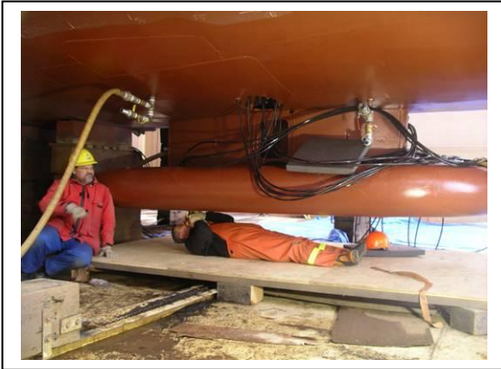
Vector, EM710 (gondola installation '09)
