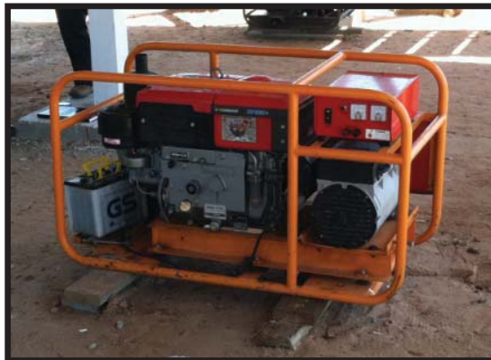
New Generator used aboard R/V SEA KING
