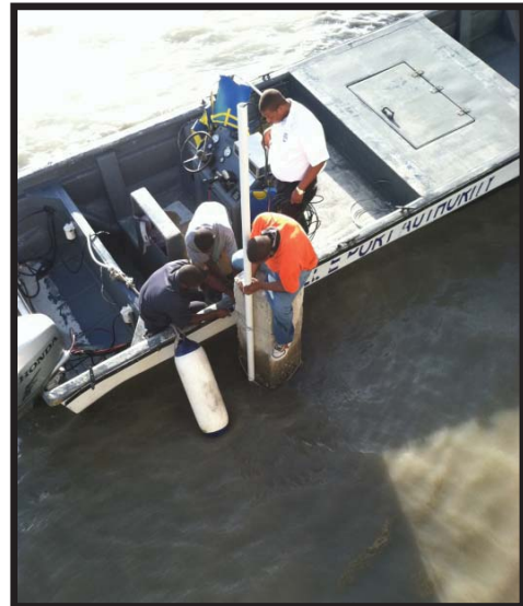
Mounting the Valeport 740 Tide Gage – Fixed to a 1-inch PVC pipe, the sensor was mounted inside a protective 3-inch PVC pipe well (left). BPA personnel strapped the well to a concrete piling near the PBL pier (right) and manually measured the distance between the sensor and top of the well to provide a leveling point to the benchmark.
