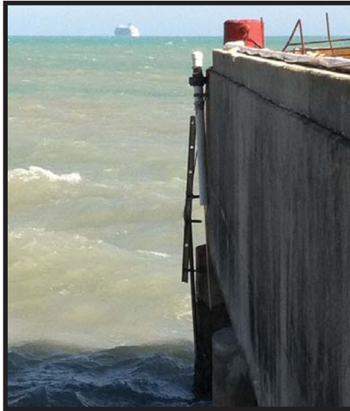
PBL Tide Gage on 22 February 2011 – The Aquatrak system appears to have sustained significant damage from storm and/or shipping activity at the pier head. The lower mounting clamp and lower sections of the outer (well) and inner (sounding tube) PVC piping have been removed.
