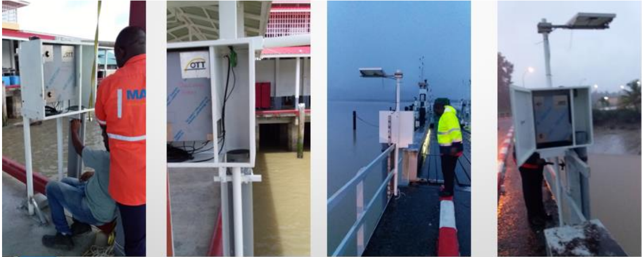
Figure 3 : Installation of OTT tide gauges with floating system
