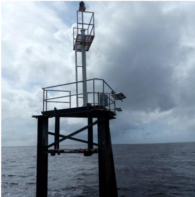
Figure 4 : Installed OTT RLS Radar Level Sensor
