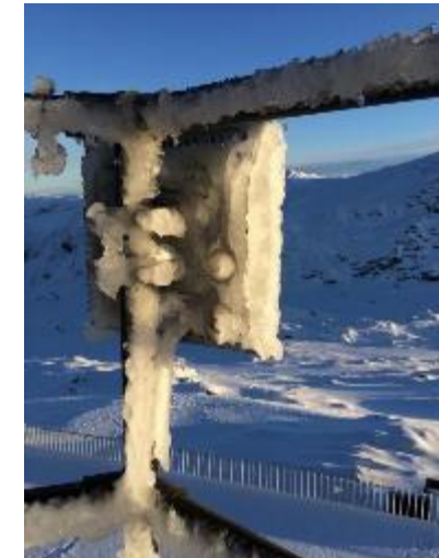
MBR 189 installed on the mountain Ulriken. (640 meter antenna height)
