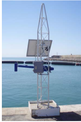
Figure 15. Radar tide gauge
