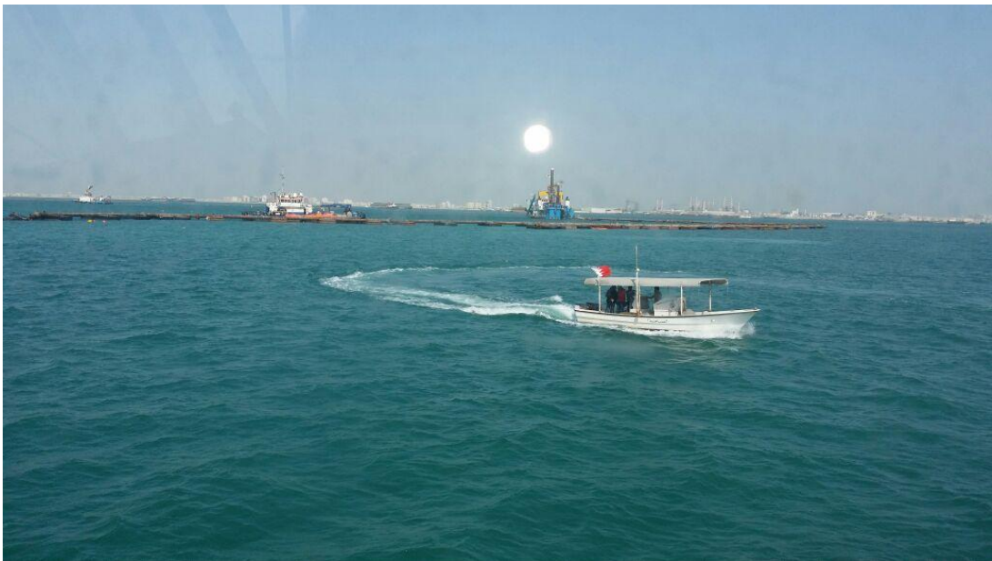
Dredging in progress for East Sitra project at the location identified by HSD
